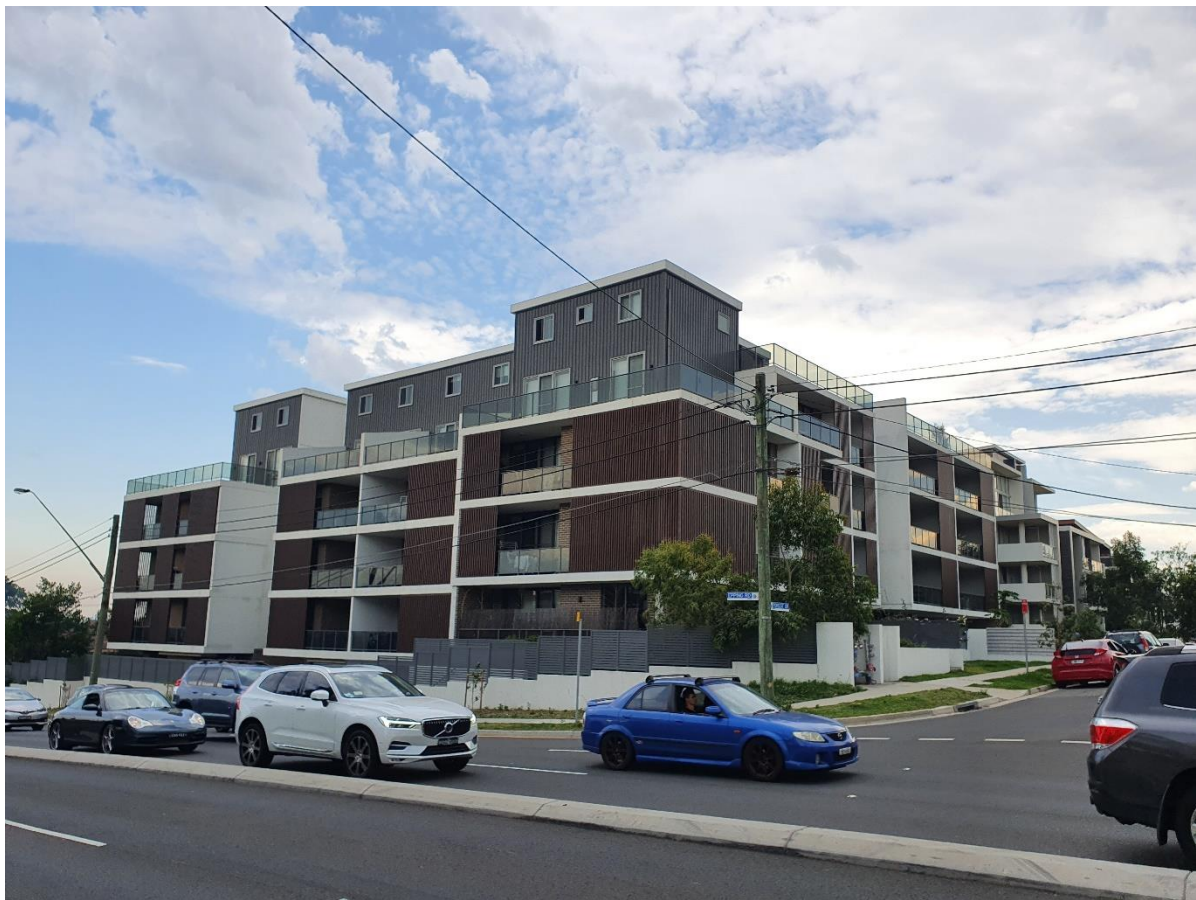
Figure 11: No. 20-24 Epping Road viewed from northern side of Epping Road
