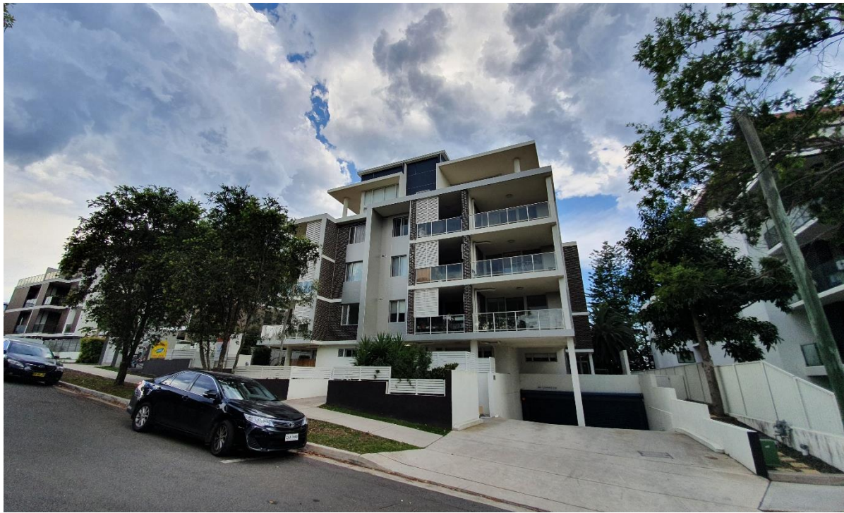
Figure 12: No. 1 Forest Grove viewed from Forest Grove
