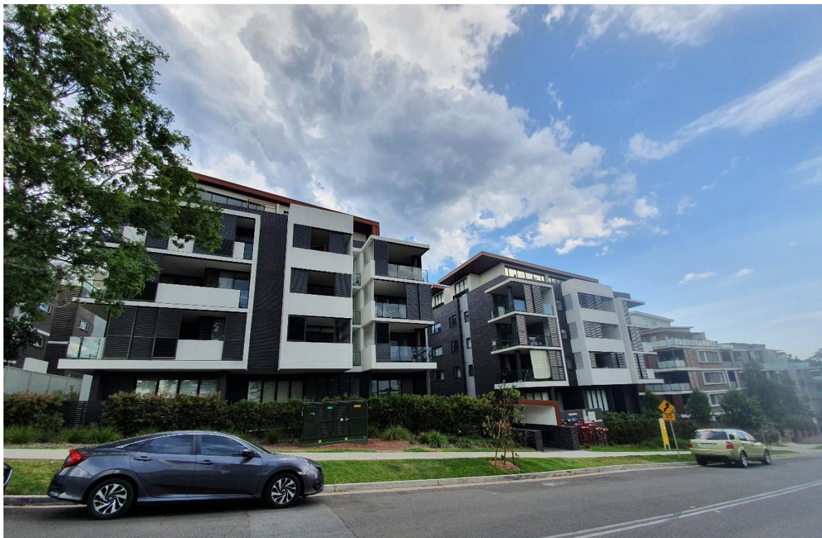
Figure 13: No. 3-7 Forest Grove viewed from Forest Grove, with further residential flat buildings within the precinct visible to the south (right-hand side)
